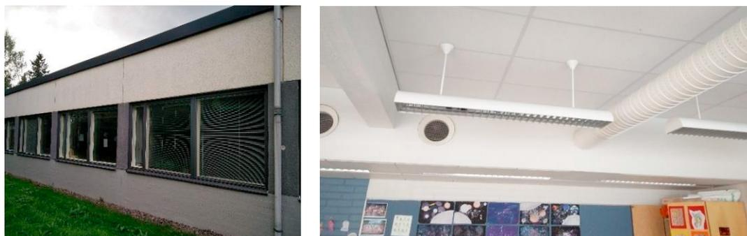
Fig. 1. (a) Studied building part; (b) A typical supply air duct diffuser and an extract air grille in a classroom.
